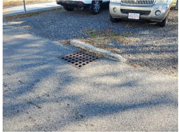
Photo 2: Catch basin on Shawsheen Rd. Three catch basins on Shawsheen Rd discharge to an outlet in Costello Park.
