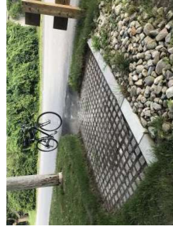
Sediment Forebay with Paver Mat and Level Spreader (Credit HW)
