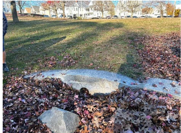
Photo 4: Granite headwall with outlet of 8-inch PVC pipe.
