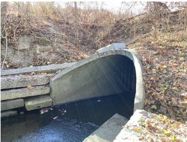
Erosion at 60-inch outfall to Shawsheen River in Lawrence
