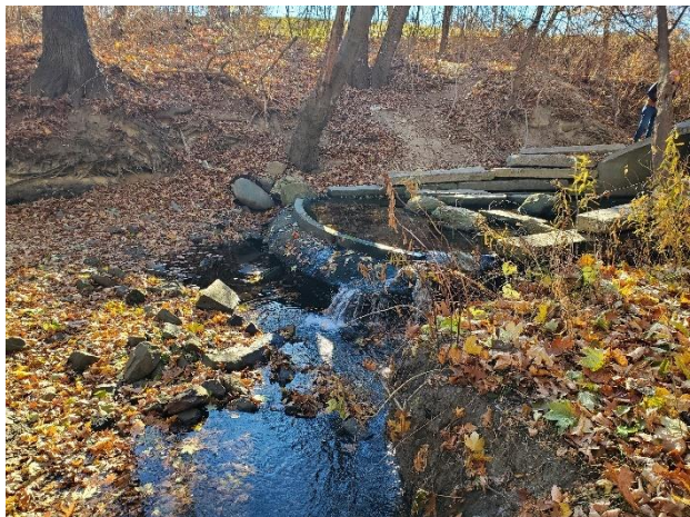
Erosion at 60-inch outfall to Shawsheen River in Lawrence
